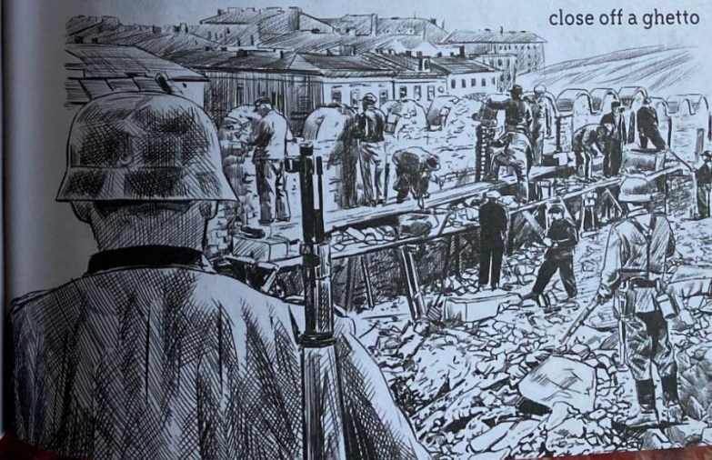
Workers build a wall to close off a ghetto
